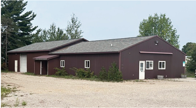
BUCKLEY 125 Industrial Drive
